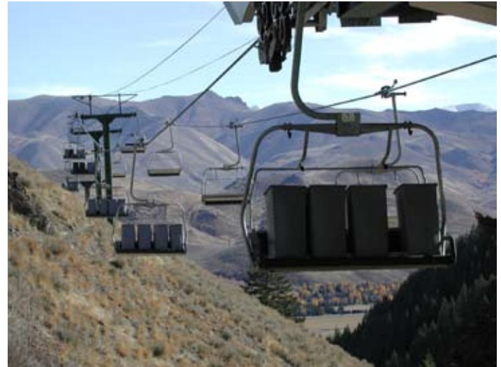
Testing a retrofit drive installation
